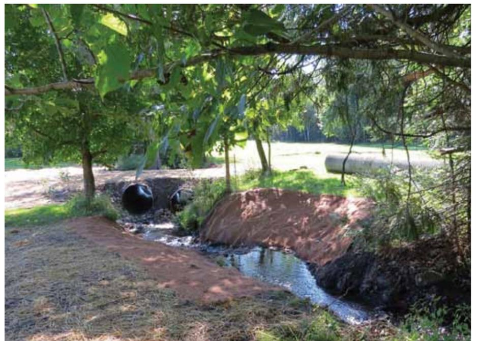
MATUSKA'S CREEK NEAR GRAND RAPIDS MINNESOTA AFTER THE RECENT CULVERT REPLACEMENT. NOTE THE DRY CULVERT ON THE LEFT DESIGNED TO HANDLE HIGH FLOW EVENTS.
