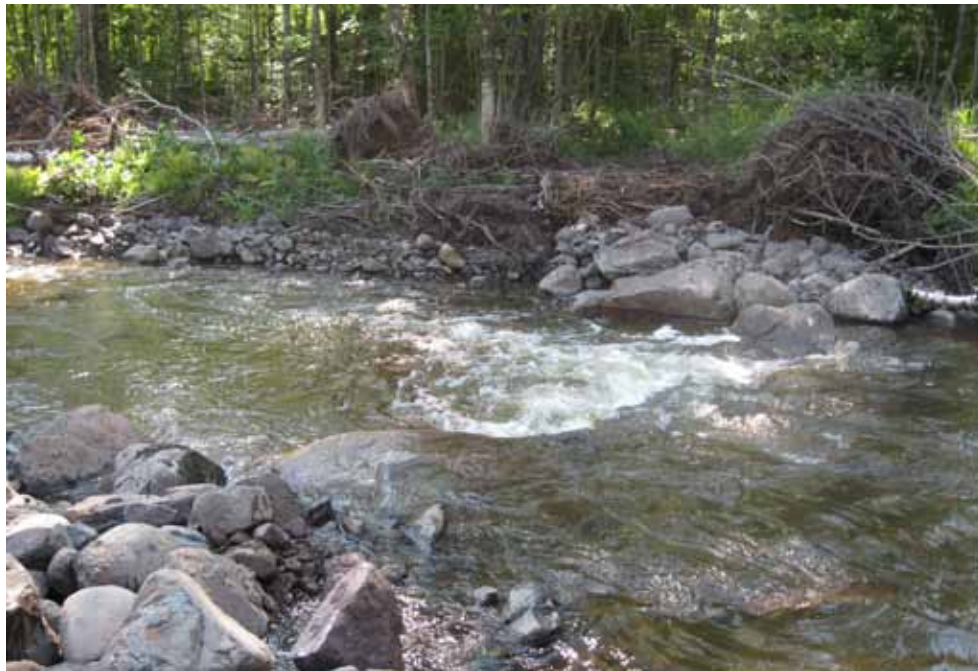
A FINISHED ROCK VEIN ON THE LOWER SUCKER RIVER PROJECT.
