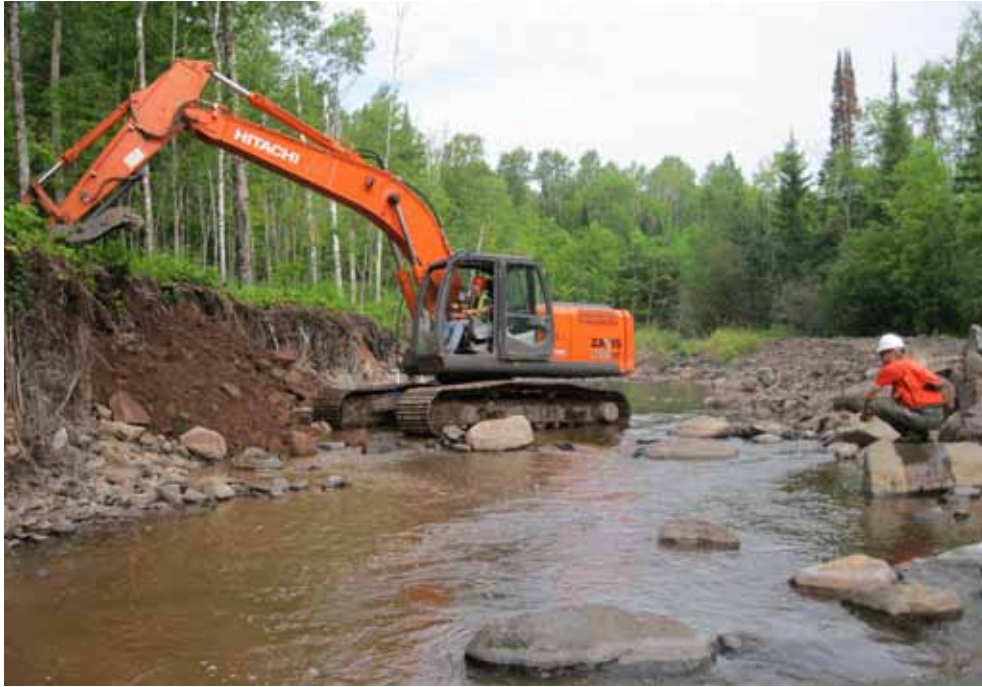
SLOPING THE BANK ON THE LOWER SUCKER RIVER PROJECT
