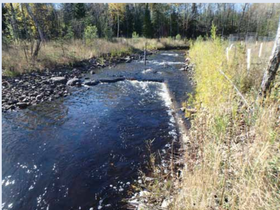
THIS J-HOOK VANE INSTALLED ON THE STEWART RIVER HIGHLIGHTS NOT ONLY THE DEPTH OF THE POOL SCoured, BUT ALSO THE EFFECTIVE VEGETATION ON THE BANK, ABLE TO GROW DUE TO PROTECTION FROM DIRECT FLOWS.
