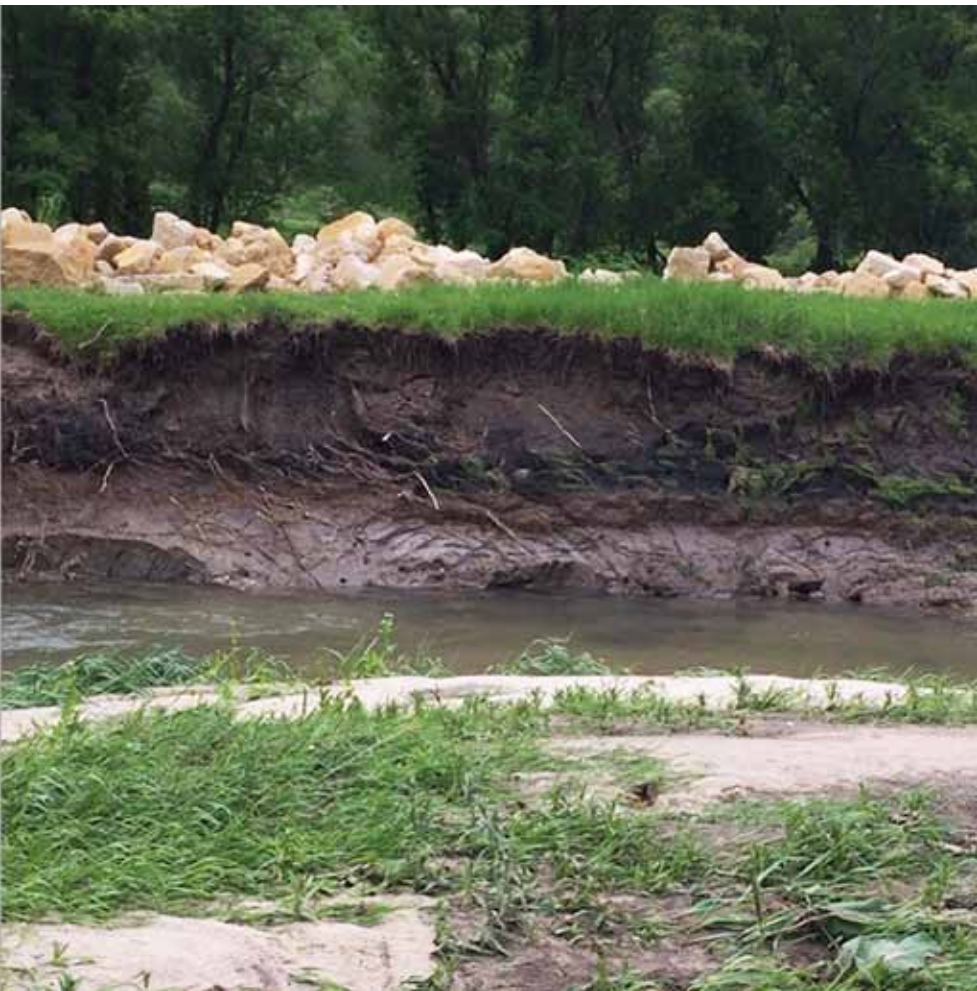
A SECTION OF GARVIN BROOK PRIOR TO RESTORATION WORK. THE BANKS WERE LATER GRADED TO GRADUAL 3:1 SLOPES, AND ROCK WAS USED TO HOLD THE SLOPE'S TOE UNTIL GRASSES TOOK HOLD. LIMESTONE ROCK SITS ON TOP OF THE BANK, READY TO USE IN THE NOW-COMPLETED PROJECT WORK.
