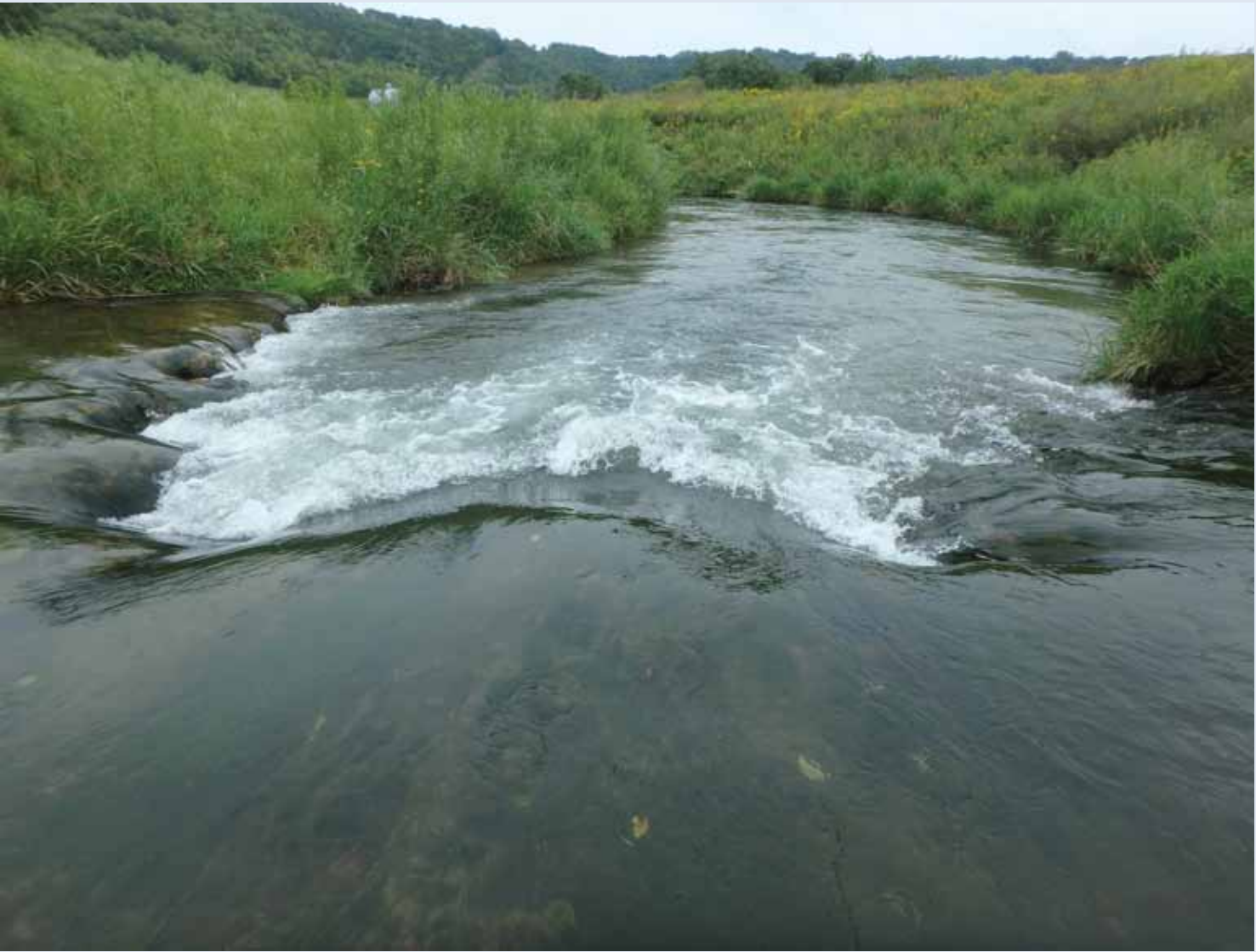
THIS ROCK CROSS VANE ON RUSH CREEK IN SE MINNESOTA DIRECTS WATER FLOWS TO THE CENTER OF THE STREAM CHANNEL, SCOURING THE AREA AND MAINTAINING POOL DEPTH FOR A LONG REACH BELOW THE STRUCTURE.
