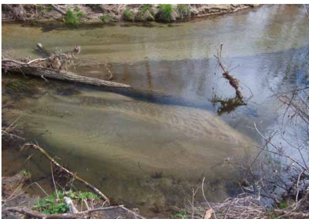
HAY CREEK PRE-PROJECT: AN OVERLY WIDE CHANNEL HAS FILLED WITH SAND, MAKING THE STREAM SHALLOW.
