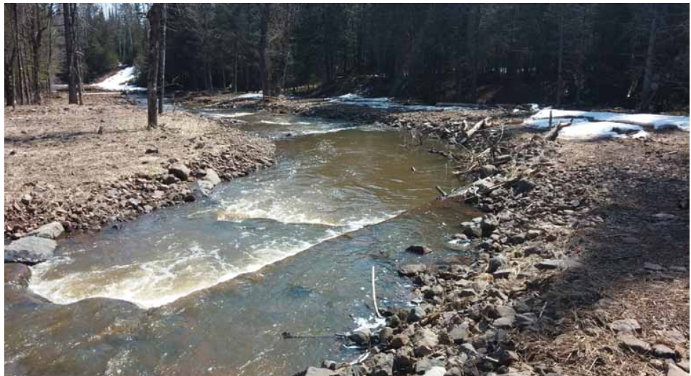
A SEVERE FLOOD FILLED THE CHANNEL OF THE LITTLE STEWART RIVER WITH ROCK AND DEBRIS IN THE PHOTO TO THE UPPER LEFT. ABOVE, THE SAME REACH IS SHOWN AFTER RESTORATION. THE STREAM HAS ACCESS TO THE NEW FLOODPLAIN IN TIMES OF HIGH WATER. ROCK AND LOG STRUCTURES DIRECT FLOWS TO THE CENTER OF THE STREAM.
