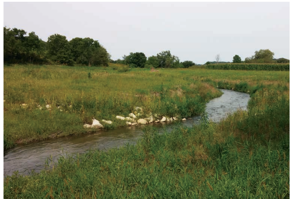
GENTLY SLOPED BANKS ARE SEEDED AND COVERED IN EROSION CONTROL FABRIC AFTER INITIAL GRADING AND CHANNEL WORK IN THE PHOTO ON THE LEFT. A YEAR LATER, NATIVE VEGETATION THRIVES IN AUGUST OF 2016 AFTER COMPLETED RESTORATION WORK ON MILL CREEK IN THE PHOTO ON THE RIGHT.
