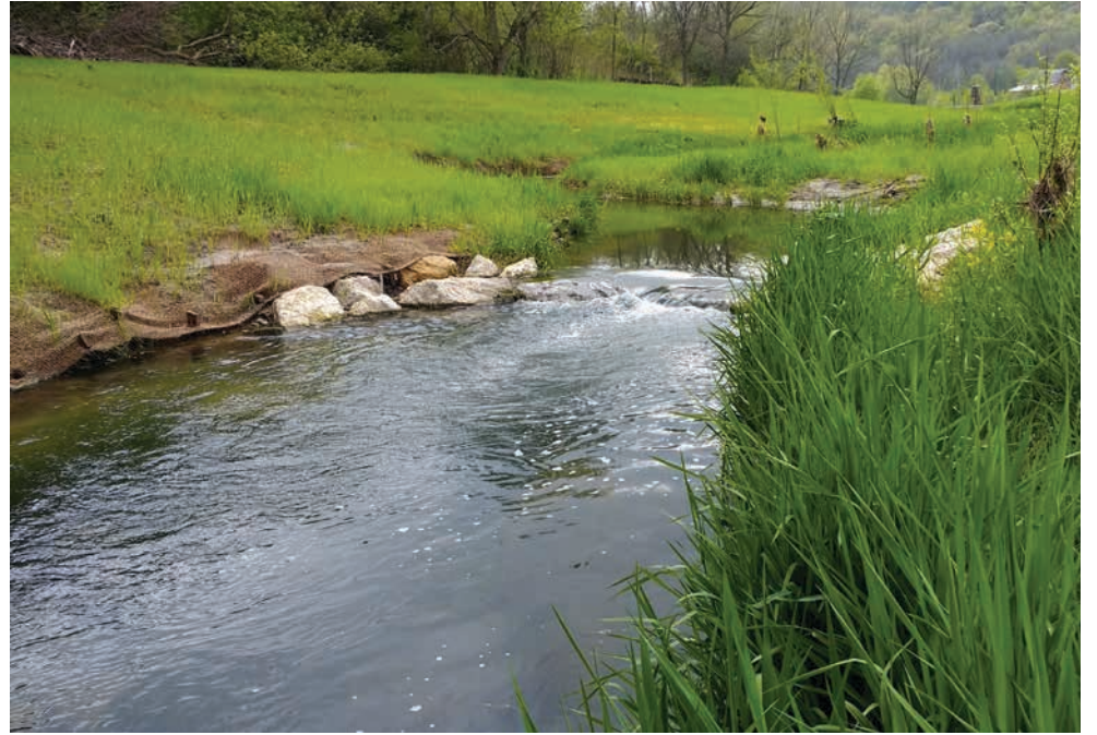
BANKS HAVE BEEN SLOPED, SEEDED AND COVERED IN EROSION CONTROL FABRIC AFTER GRADING AND CHANNEL WORK (LEFT). AFTER WINTER, SPRING VEGETATION THRIVES IN MAY OF 2017 IN COMPLETED RESTORATION WORK ON EAST INDIAN CREEK (RIGHT).
