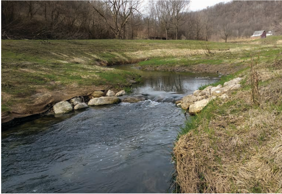
BANKS HAVE BEEN SLOPED, SEEDED AND COVERED IN EROSION CONTROL FABRIC AFTER GRADING AND CHANNEL WORK (LEFT). AFTER WINTER, SPRING VEGETATION THRIVES IN MAY OF 2017 IN COMPLETED RESTORATION WORK ON EAST INDIAN CREEK (RIGHT).
