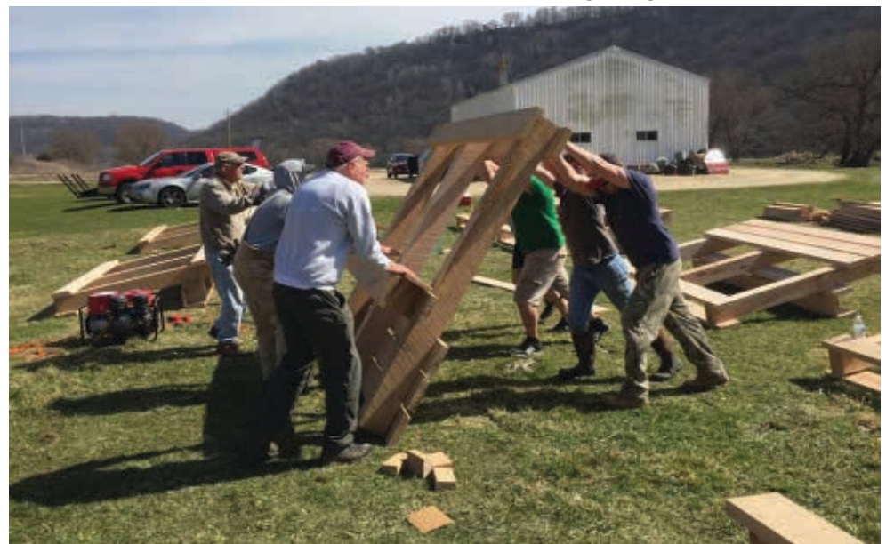
WIN-CRES TU CHAPTER VOLUNTEERS CONSTRUCT HABITAT STRUCTURES
