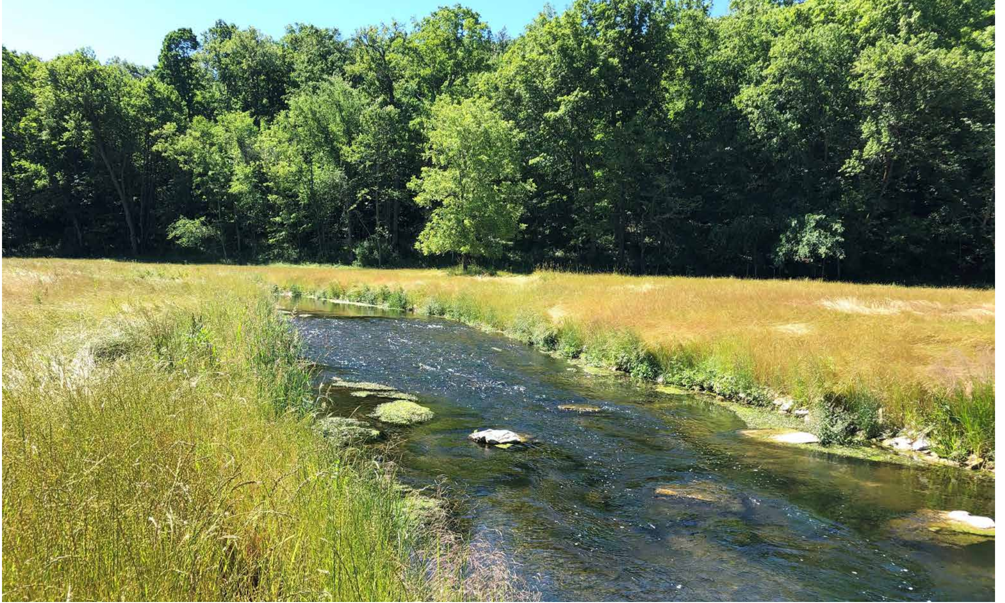
WISEL CREEK HABITAT RESTORATION NEARS COMPLETION AS VEGETATION BECOMES ESTABLISHED.
