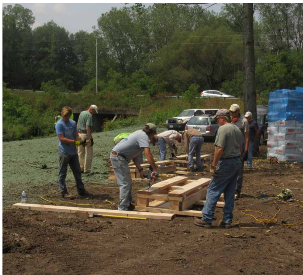
MEMBERS OF THE WIN-CRES CHAPTER BUILD A LUNKER STRUCTURE FOR THE RECENT UPPER RUSH CREEK HABITAT IMPROVEMENT PROJECT
