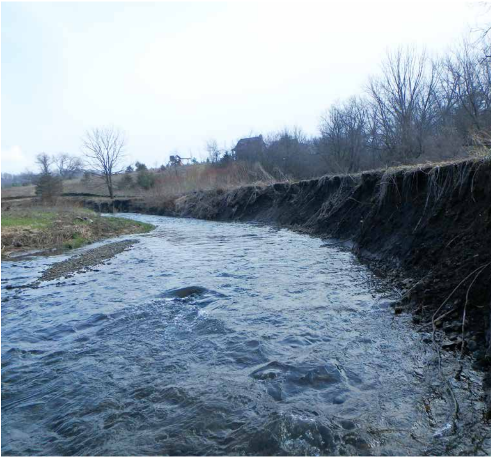
ERODING BANKS ON WISEL CREEK WERE EXCAVATED TO RESTORE THE FLOODPLAIN, HALT EROSION AND IMPROVE IN-STREAM HABITAT.
