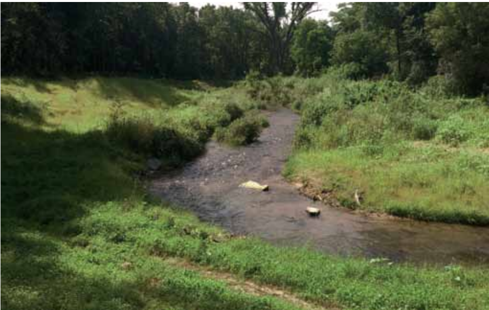
THIS BANK ON LEFT SIDE OF HAY CREEK HAS A BANKFULL BENCH BUILT OUT 20 FEET FROM A TALL, VERTICAL ERODING BANK. THE FORMER BANK EDGE WAS WHERE THE NEW GRASSY SLOPE MEETS THE TREE LINE.
