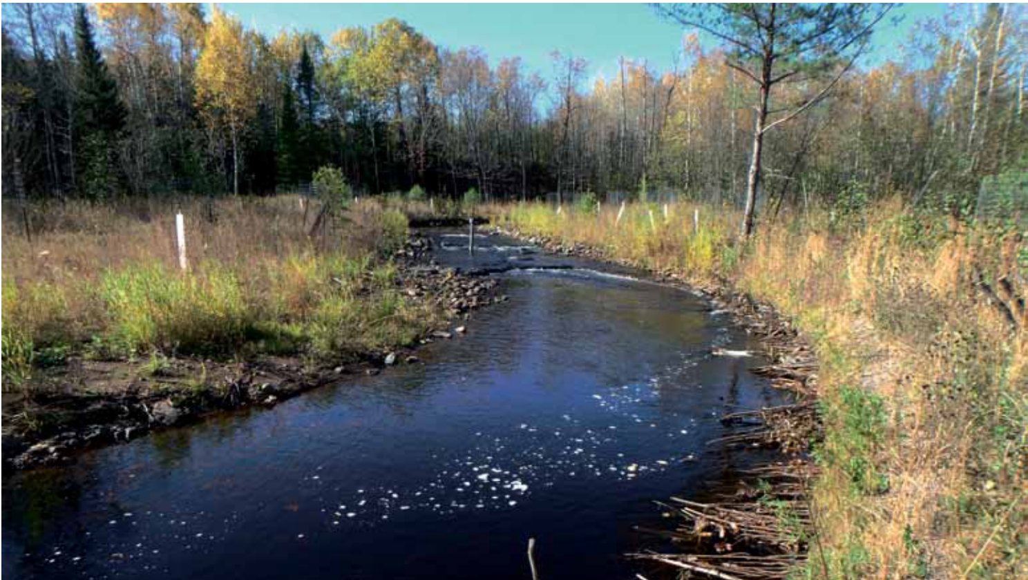
TOE WOOD ON THE STEWART RIVER WILL DISSIPATE ENERGY OF HIGHER FLOW, KEEPING BANK FROM ERODING. BROOK TROUT TAKE UP FEEDING LINES UNDER FOAM LINE IN PICTURE, ADJACENT TO COVER PROVIDED BY SUBMERGED WOODY HABITAT.
