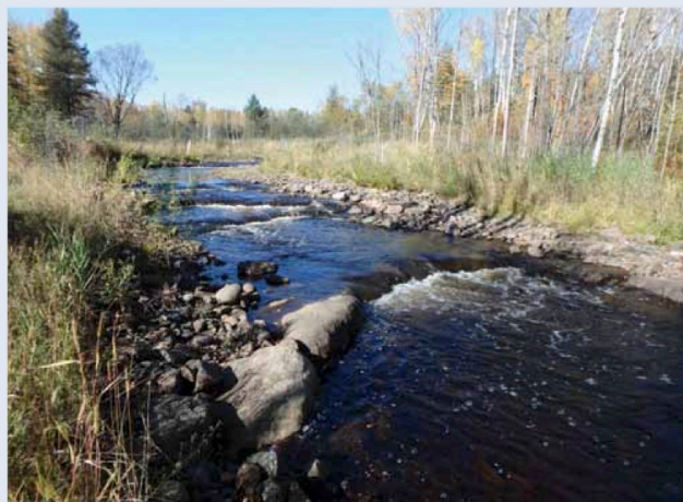
THIS SERIES OF ROCK VANES IN THE STEWART RIVER HELP MAINTAIN GRADE CONTROL WHILE KEEPING DEEP POOLS SCOURED. THESE POOLS ARE VITAL FOR SEDIMENT TRANSPORT IN ADDITION TO PROVIDING GREAT TROUT HABITAT.
