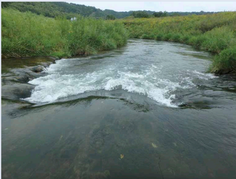
THIS ROCK CROSS VANE ON RUSH CREEK IN SE MINNESOTA DIRECTS WATER FLOWS TO THE CENTER OF THE STREAM CHANNEL, SCOURING THE AREA AND MAINTAINING POOL DEPTH FOR A LONG REACH BELOW THE STRUCTURE.
