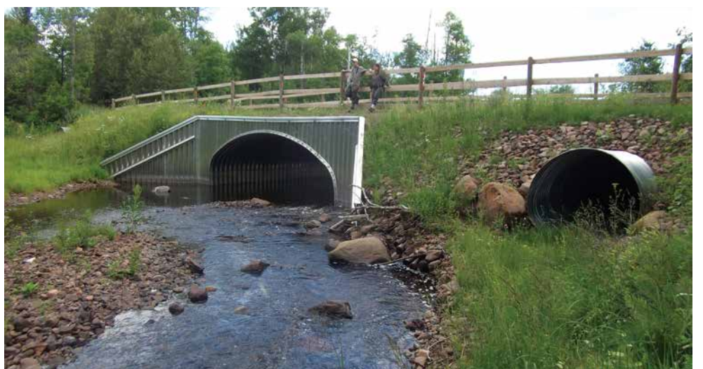
TOP: PERCHED CULVERTS PREVENT BROOK TROUT IN THE BAPTISM RIVER FROM ACCESSING 30 MILES OF GOOD HABITAT. PHOTO COURTESY OF FINLAND AREA FISHERIES OFFICE.
