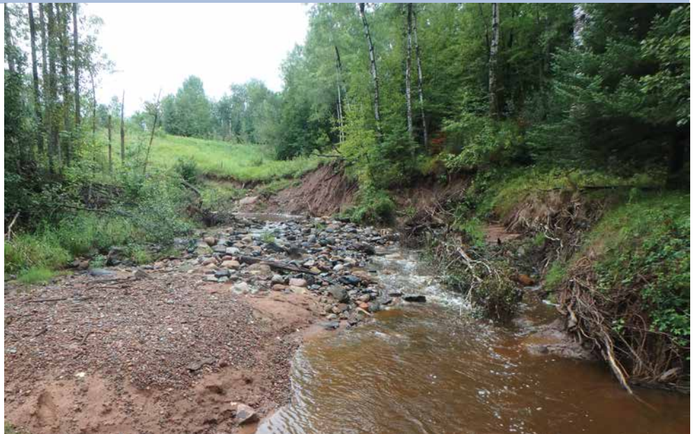
LOOKING UPSTREAM ON A NEMADJI RIVER TRIBUTARY TOWARD A ROAD WITH AN UNDERSIZED CULVERT. THE MASSIVE SIZE OF THIS ROADWAY/DAM BUILT ACROSS THE VALLEY IS VISIBLE. THE CULVERT CONSTRICTS FLOOD FLOWS, CREATING A MASSIVE "FIRE HOSE" EFFECT, BLOWING OUT THE BANKS IN THE FOREGROUND.
