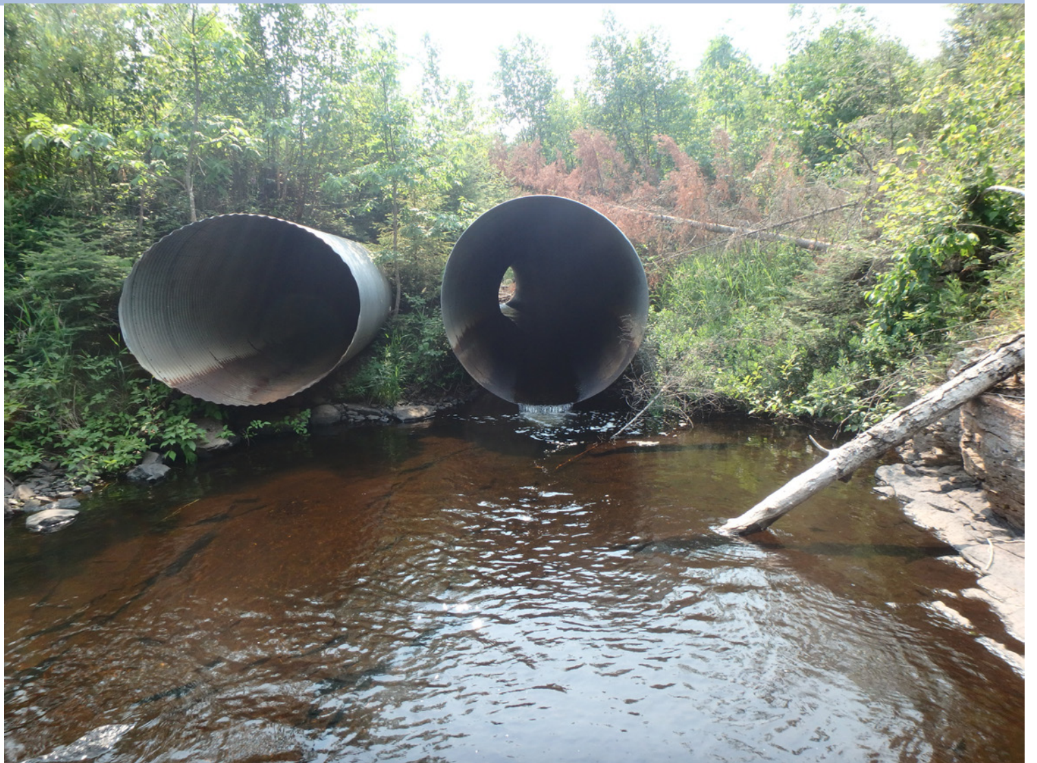
PERCHED CULVERTS PREVENT BROOK TROUT IN THE BAPTISM RIVER FROM ACCESSING 30 MILES OF QUALITY HABITAT.
