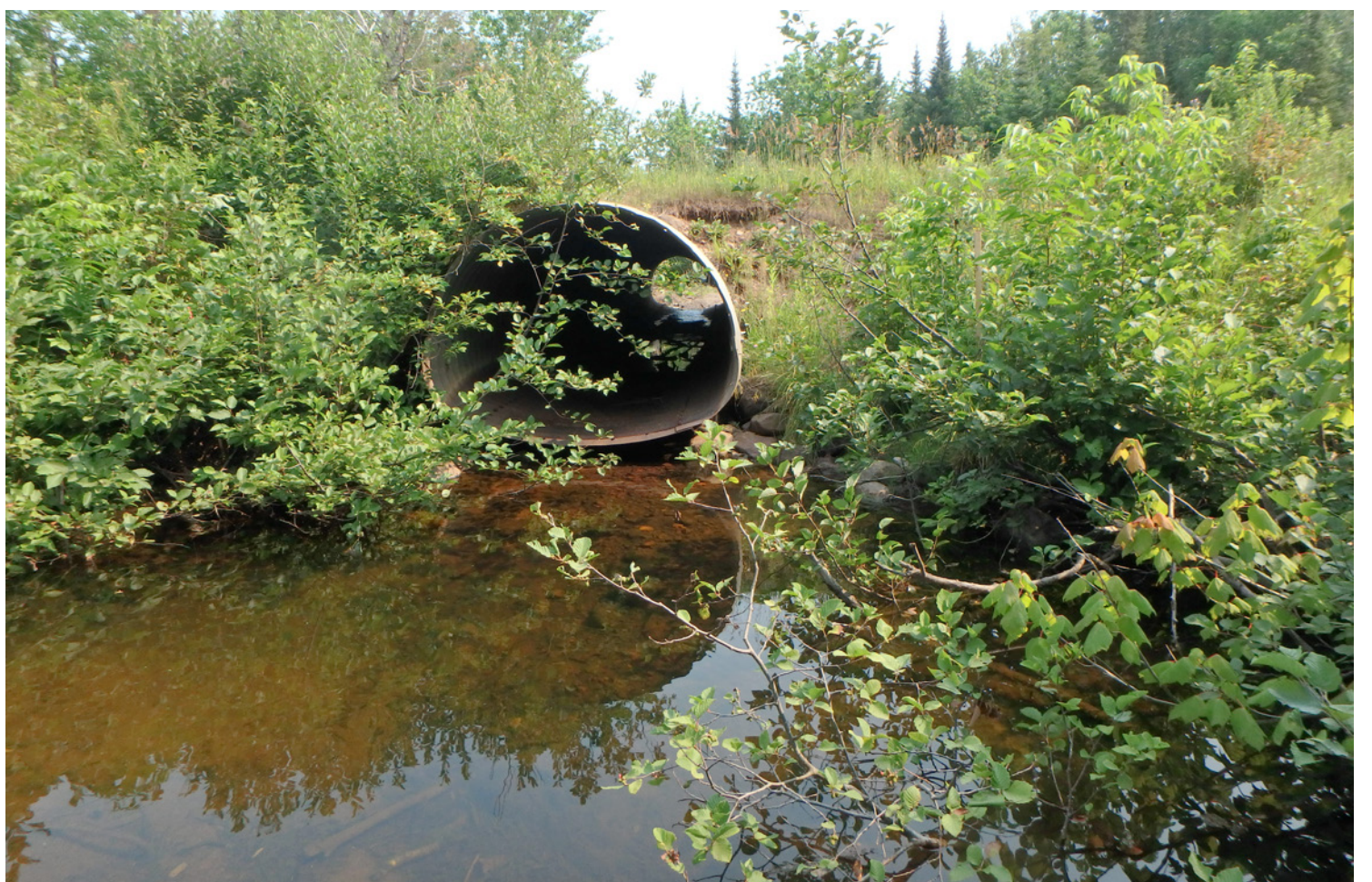
THIS CULVERT ON A COLDWATER TRIBUTARY TO THE TWO ISLAND RIVER BLOCKS FISH PASSAGE.
