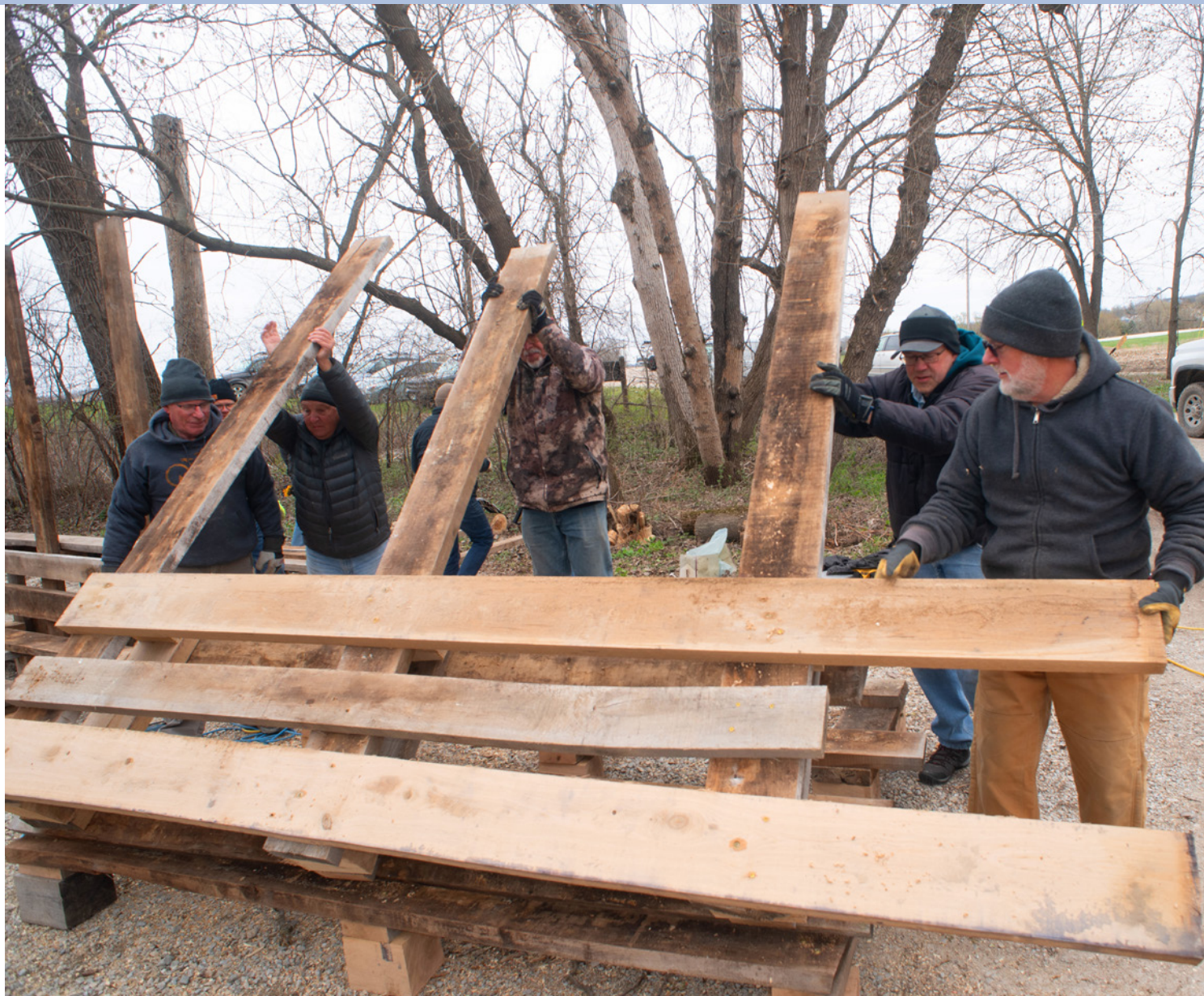
VOLUNTEERS HEAVE A LUNKER STRUCTURE TO BE INSTALLED IN MILL CREEK. THESE PROVIDE DEEP COVER FOR FISH, AS WELL AS ADDED STREAMBANK STABILITY.
