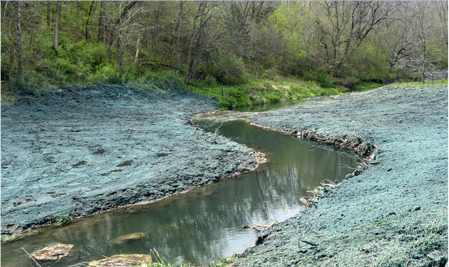
A NEWLY RESTORED REACH ON RICE CREEK WITH A THICK COAT OF HYDROMULCH TO HOLD SOIL AS COVER CROP GROWS IN (MAY 2024).
