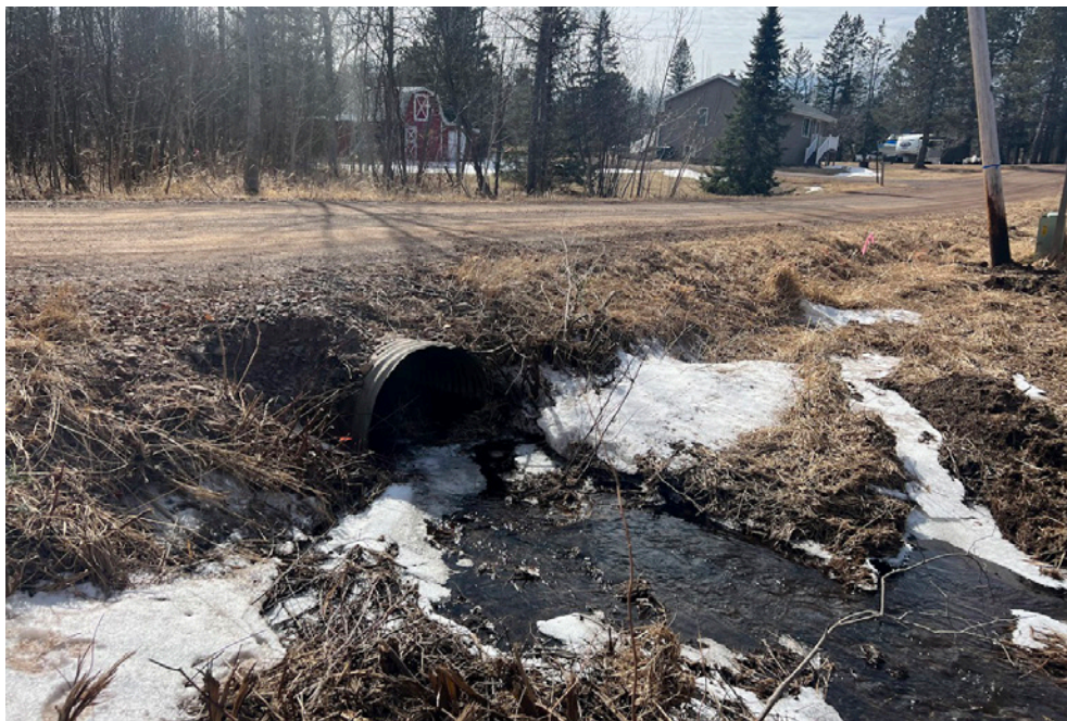
BAPTISM RIVER TRIBUTARY BARRIER CULVERT PRE-REPLACEMENT (LEFT) AND POST-REPLACEMENT (RIGHT) IN FINLAND, MN. A SINGLE UNDERSIZED CULVERT WAS REPLACED WITH TWO METAL ARCHED CULVERTS, INCLUDING A LOW FLOW AND HIGH FLOW CULVERT.
