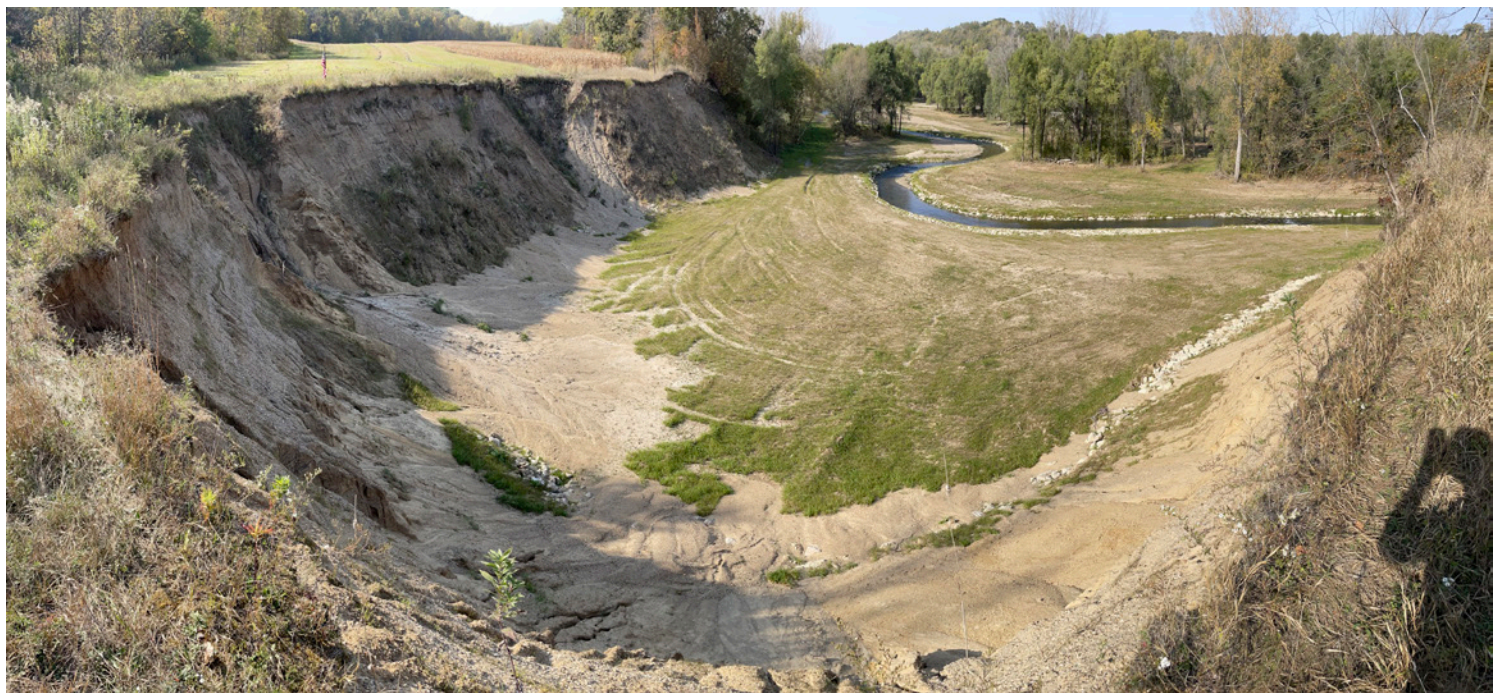
TOP: MAZEPPA PRE-PROJECT, STREAM CHANNEL AGAINST A STEEP ERODING BLUFF. (PHOTO: DUSTY HOFFMAN, MN DNR) BOTTOM: POST-PROJECT, STREAM CHANNEL PULLED AWAY FROM ERODING CLIFF. (PHOTO: DUSTY HOFFMAN, MN DNR)
