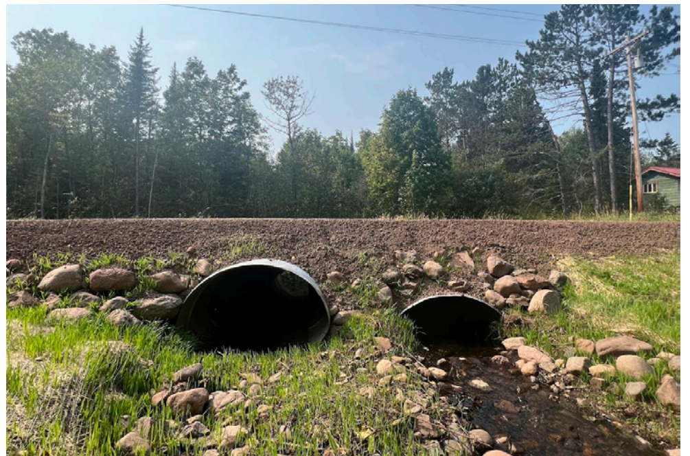
BAPTISM RIVER TRIBUTARY BARRIER CULVERT PRE-REPLACEMENT (LEFT) AND POST-REPLACEMENT (RIGHT) IN FINLAND, MN. A SINGLE UNDERSIZED CULVERT WAS REPLACED WITH TWO METAL ARCHED CULVERTS, INCLUDING A LOW FLOW AND HIGH FLOW CULVERT.
