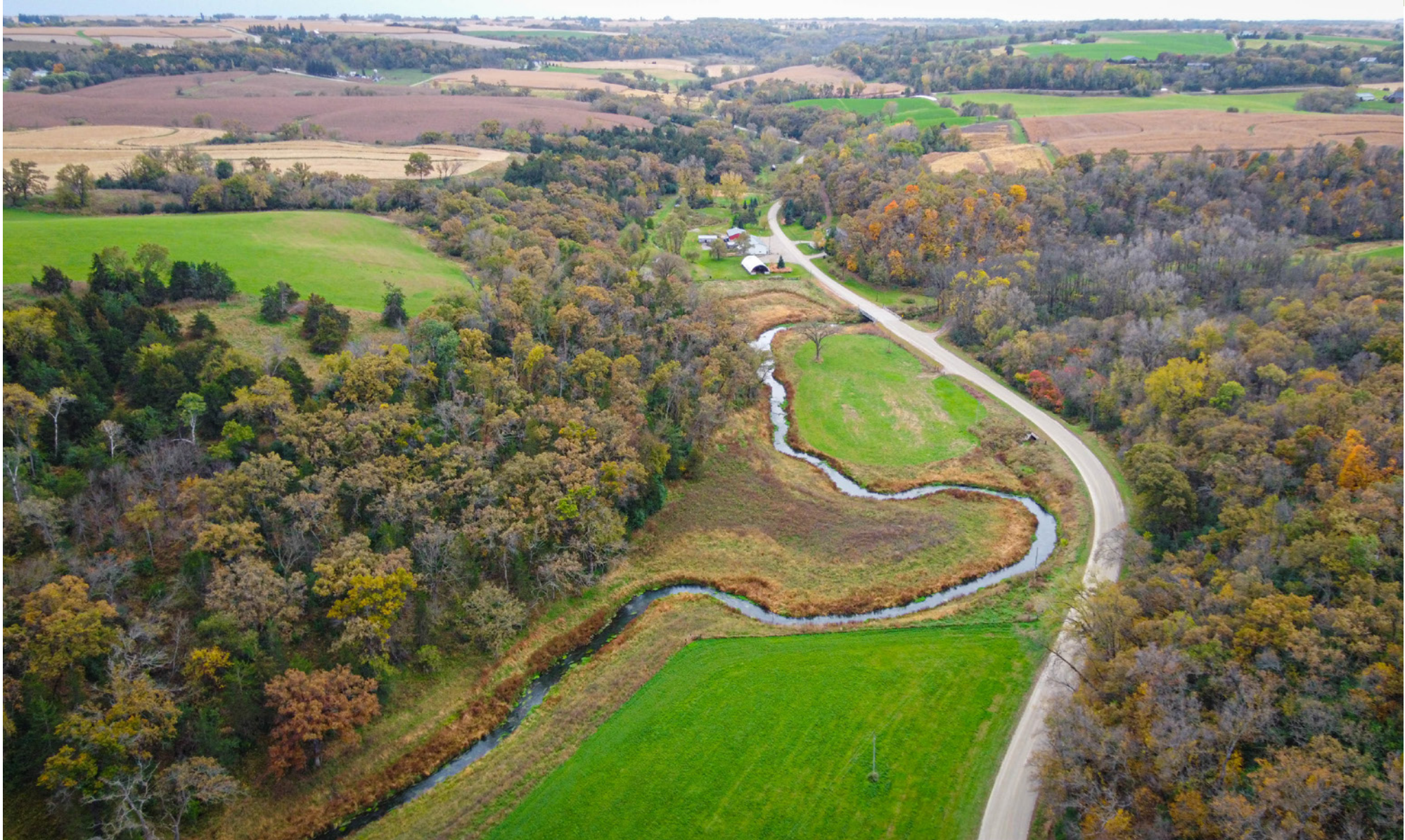
PART OF THE RICE CREEK HABITAT IMPROVEMENT PROJECT, OCTOBER 14, 2025.
